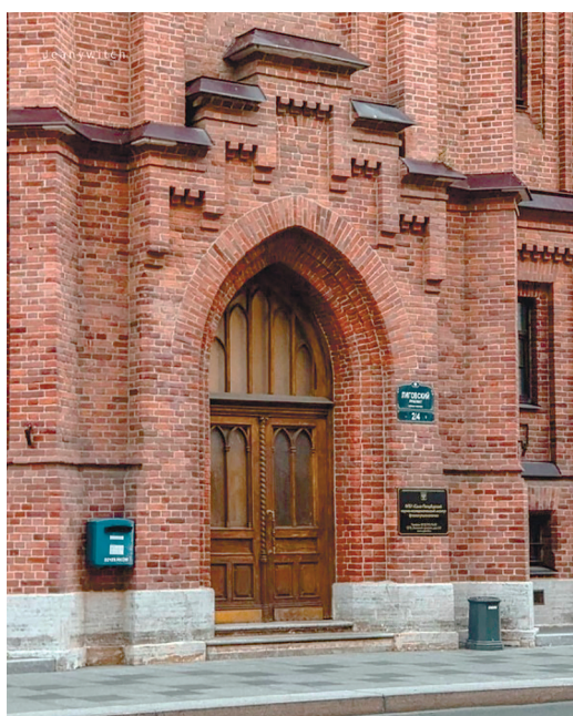
Fig. 5. Evangelical Women's Hospital. Facade elements. Main entrance [57]
